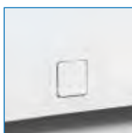
- Esgoto - Defrost drain
